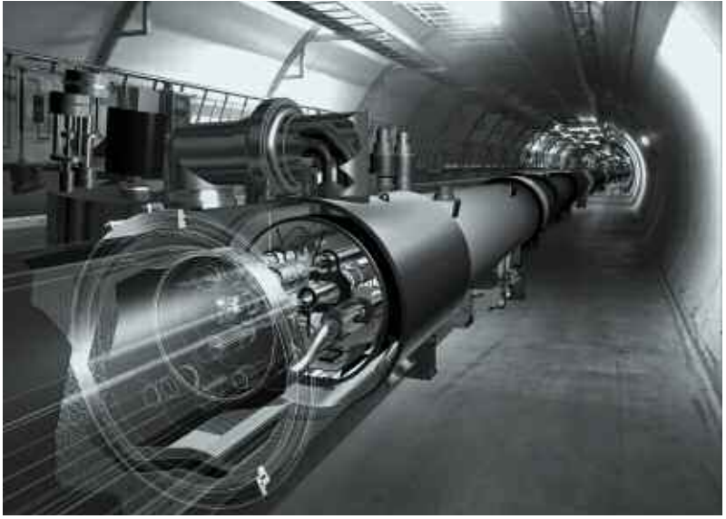
A mock-up of the LHC tunnel at CERN showing the two beam pipes in which the 7 TeV proton beams will travel around the 27-km ring.
