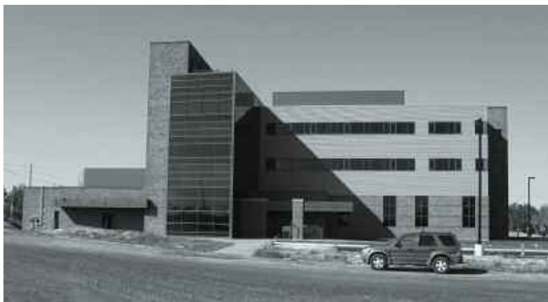
The new surface building of the SNOLab facility near Sudbury, housing offices, meeting rooms, and laboratory space.
