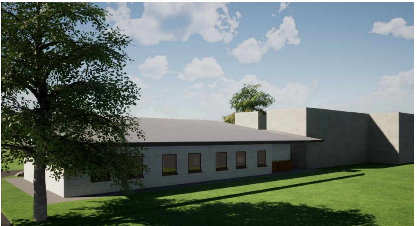
Rear view of TIP building
