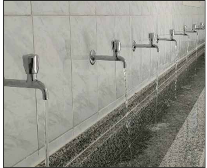
Newly installed potable water general access points.
