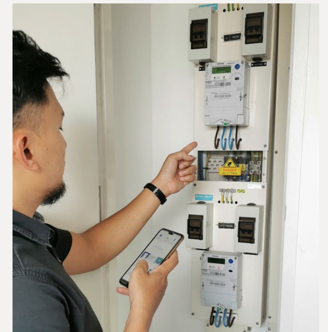
Advanced electricity meters enable households to track their half-hourly electricity consumption via the SP Utilities mobile app.
