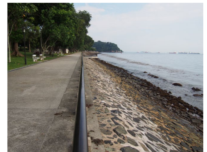
Sloping revetment at Labrador Nature Reserve. A revetment is a sloping structure built to absorb the energy of incoming waves and prevent coastal erosion.
