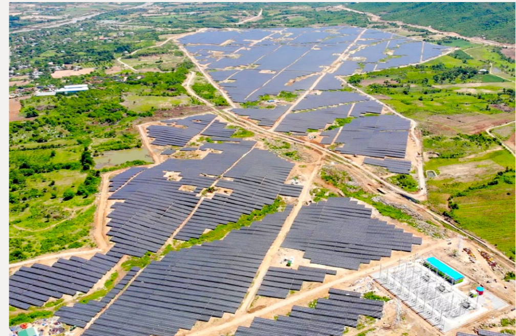
Sunseap's 168 MWp solar farm in Ninh Thuan, Vietnam is one of the largest in the country. Sunseap and InfraCo Asia contributed three billion Vietnamese dong (S$173,749) to fund the construction of concrete roads surrounding the site. At peak construction period, the project created over 2,000 jobs, mostly for locals in the area.
