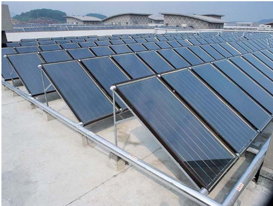
Figure 1.5: Flat plate solar collectors photo
