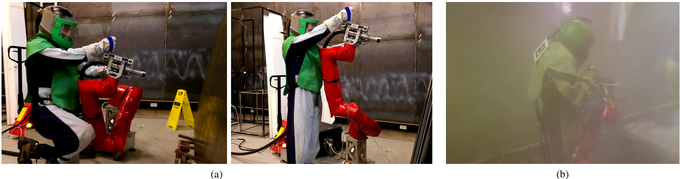
Fig. 10. (a) The ANBOT tested in laboratory conditions in preparation for site trials. (b) The ANBOT being used by an experience worker to perform real abrasive blasting during a site trial.
