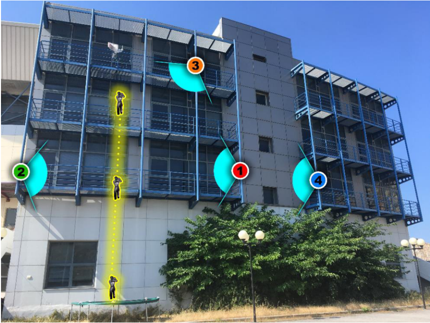
Figure 3. The four locations of the building that the optical sensor was placed, during the data acquisition experiments.
