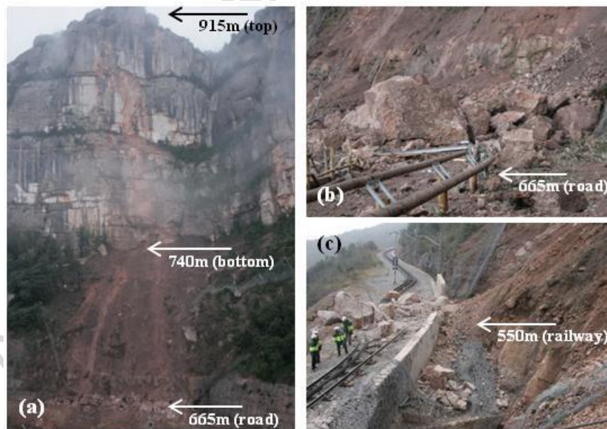
Figure 3. 28 December 2008 rockfall event of 890 m 3 at Degotalls cliff (a). In the left-hand pictures, the impacts on the road (b) and the railway (c) can be appreciated. Elevations are annotated in m.a.s.l.
