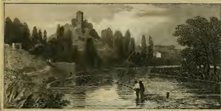
L'Assa Tower Gloucester in the distance.
