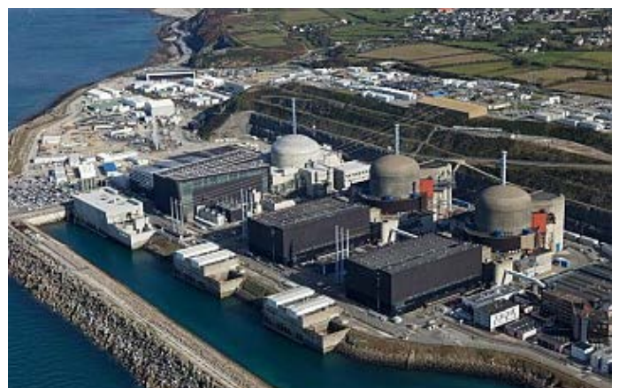
Fig. F Flammanville 3 in north-western France
