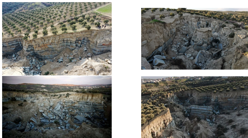
FIGURE 14. The 2023 Turkey-Syria earthquake created a canyon 35 meters deep and 200 meters wide. It could be a land subsidence from the collapse of a very deep and very large cavity formed by an underground nuclear explosion.
