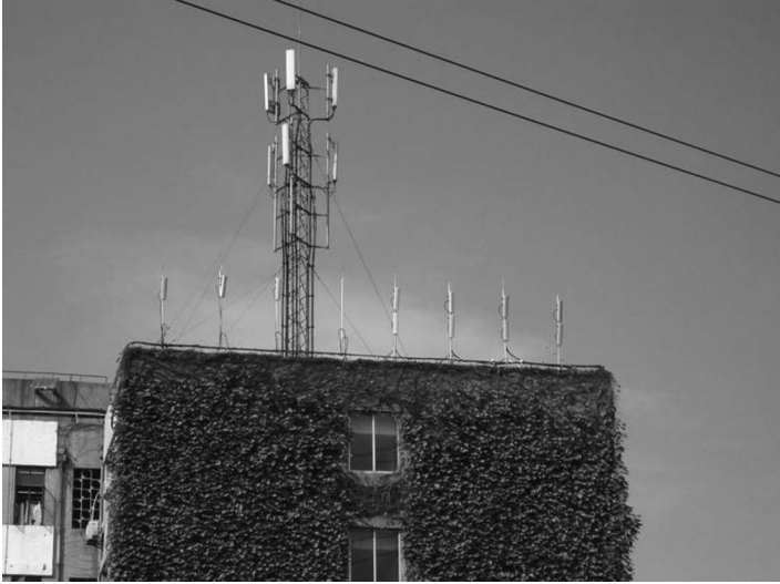
Figure 2.12 The hardware and antenna unit in the FuTURE TDD trial system.
