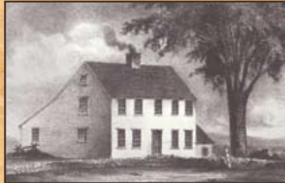
First framed house
