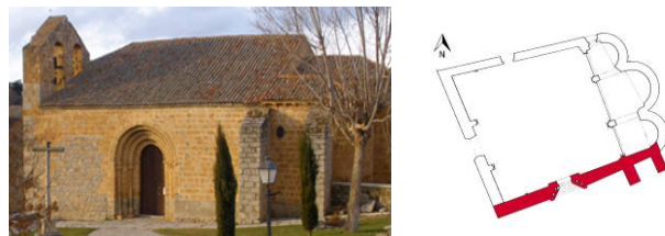
Figure 3. South façade of the Church of San Segundo in Ávila (Spain).
