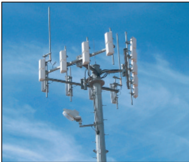
FIGURE 2.8: Sectorized cellular network employing three sectors, each one covering 120^\circ field of view.
