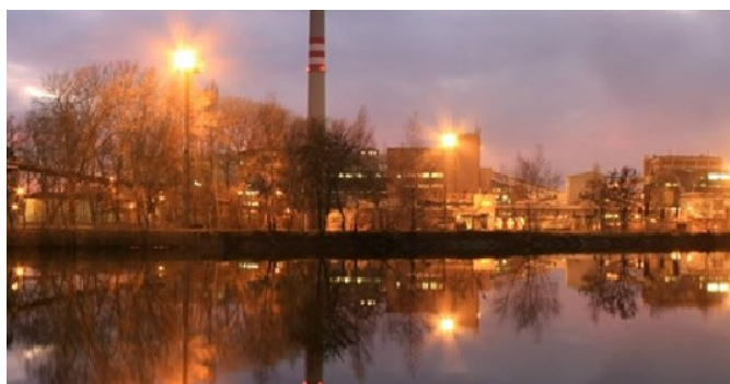
Fig. 1. Coal heating plant in the Czech Republic [UE, 2013]
