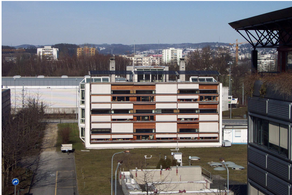
Figure 3.1: The LESO solar experimental building in Lausanne, Switzerland.
