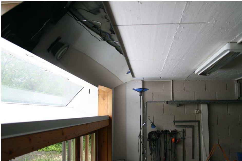
Figure 3.2: The anidolic system of mirrors that redistribute daylight in LESO's workshop.
