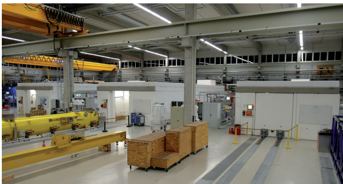
Fig. 9 Three cryomodule test benches at AMTF hall under construction.
