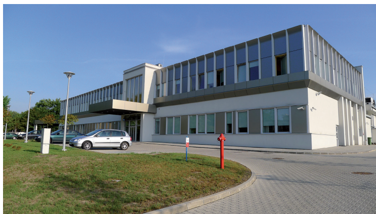
Fig. 4 Overall view of the completed CCB building ( April 2014).
