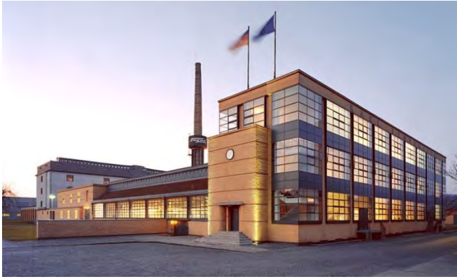
Figure 2.7 Fagus Factory (1911-13) by Walter Gropius and Adolf Meyer demonstrates the idea of the curtain wall and its freedom from load-bearing functions.
