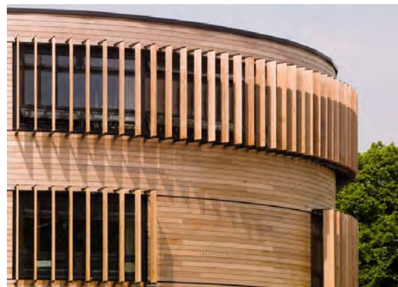
Figure 2.15 Vertical fins attached to the curved building face, Langley Academy, England.
