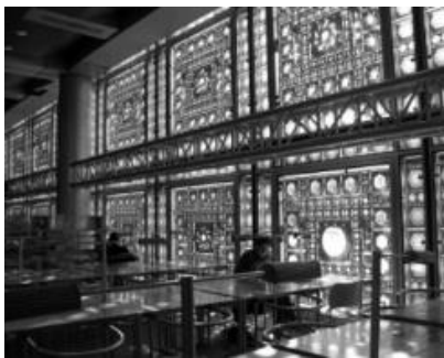
Figure 1. AWI kinetic façade system.
