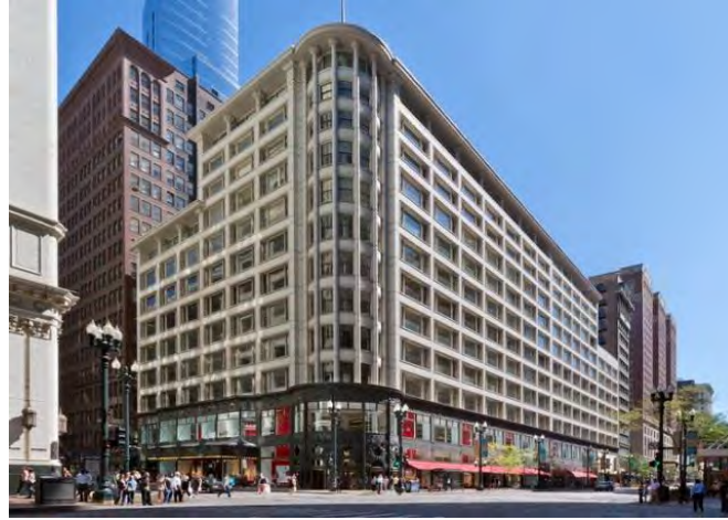
Figure 2.6 Carson, Pirie, Scott Building (1899) by Louis Sullivan offers a clear distinction between structural and non-structural elements of the facade.
