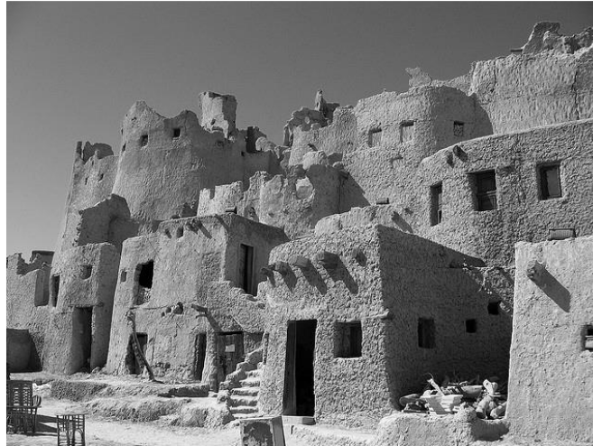
Figure 2.13 Ancient homes of Egypt with small openings
