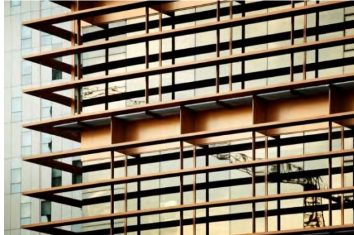
Figure 2.14 The use of horizontal shading devices in the Head Office building of Telecommunications Market Commission (CMT), Barcelona, Spain.
