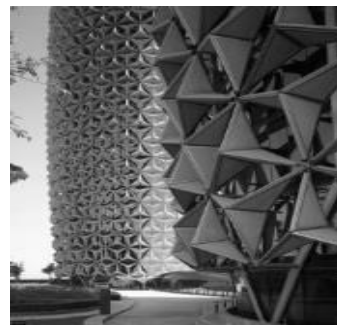
Figure 2. Al Bahar Towers
