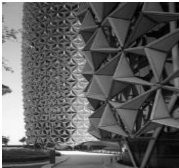
Figure 3.14 Al Bahar Towers
