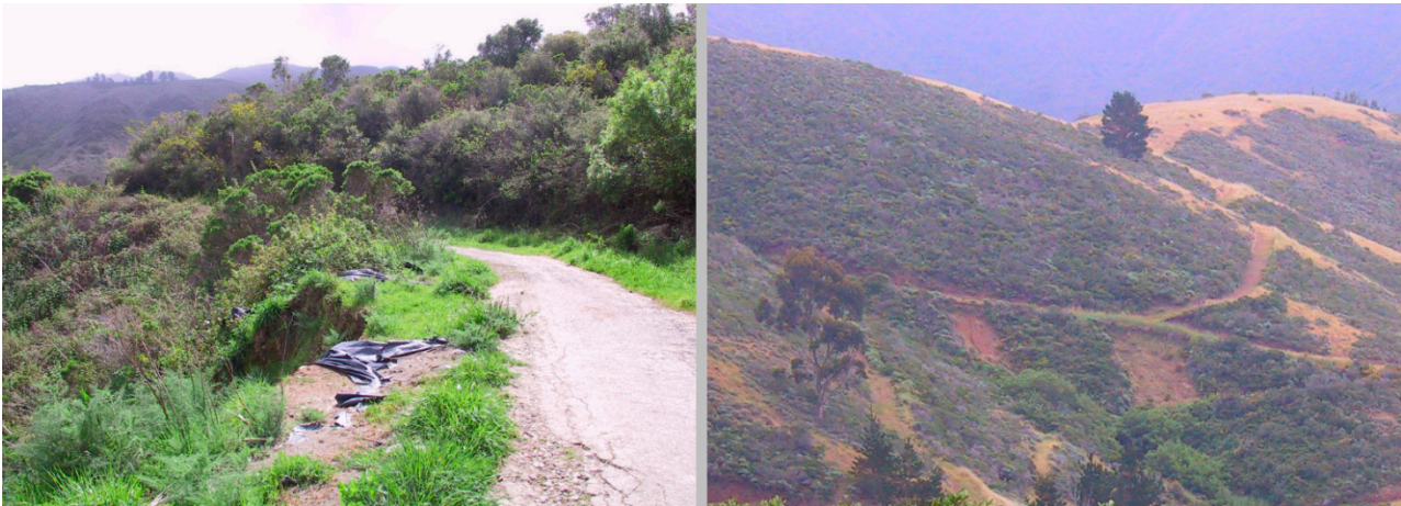
Figure 4. Shallow landslides associated with impervious runoff in San Pedro Creek watershed. At left is the crest of a failure that occurred below Higgins Road in 2003; at right are older scars from the 1970's below a dirt road above Picardo Ranch. (Photographs by Jerry Davis)
