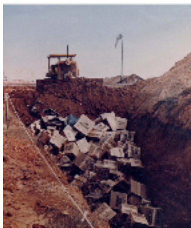
Figure 3. An example of one of the inferior waste management practices by the U.S. Department of Energy prior to 1985 associated with the widespread dispersal of radioactive waste contamination on and off the Savannah River Site, SC; similar mismanagement practices occurred at Hanford, WA. Reflective of this photo, 95% of all of Department of Energy’s (DOE’s) solid military radioactive wastes were disposed in open soil pits inside of cardboard boxes; they often sat in the pits uncovered for months at a time during all weather conditions (public photo by DOE).
