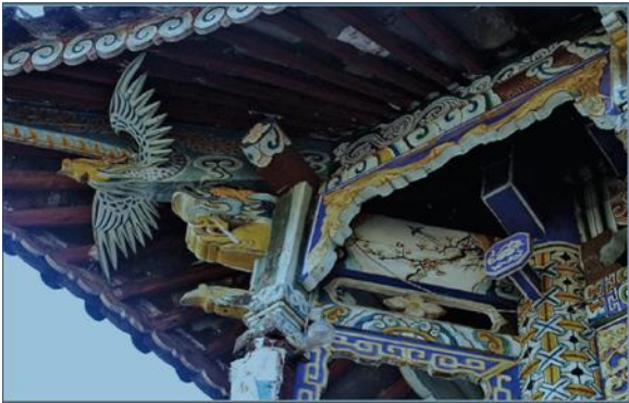
FIGURE 29: RESTORATION OF THEATRE STAGE CEILING
