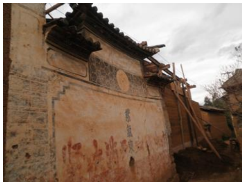
FIGURE 30: RESTORATION OF OLD HOUSES
