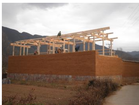
FIGURE 31: TRADITIONAL HOUSE BUILDING: STONE FOUNDATION, MUD BRICK WALLS AND WOODEN BEAMS
