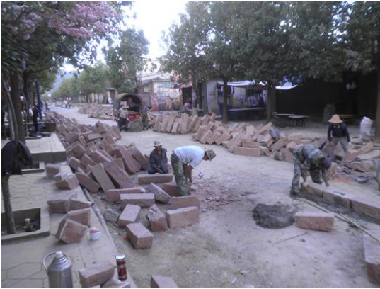
FIGURE 39: REPAVING THE MAIN ROAD IN SHAXI
