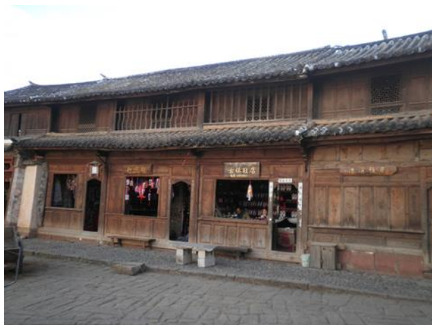
FIGURE 28: RESTORED SHOP FRONT IN SHAXI MARKET PLACE
