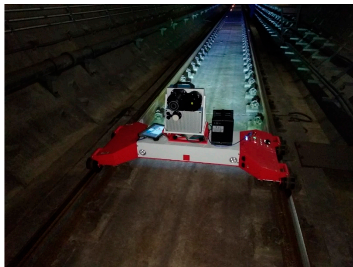
Figure 10. Tunnel scanning site.
