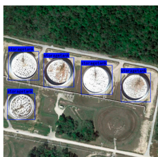
(e) storage tank
