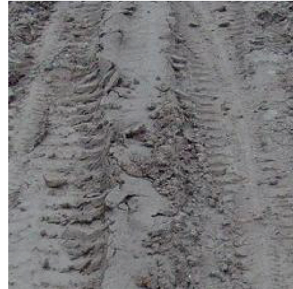
FIGURE 7: Image of mud pavement after preprocessing.
