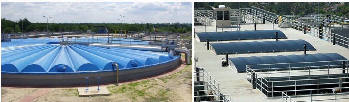
Figure 19: Examples of covered wastewater treatment tanks
