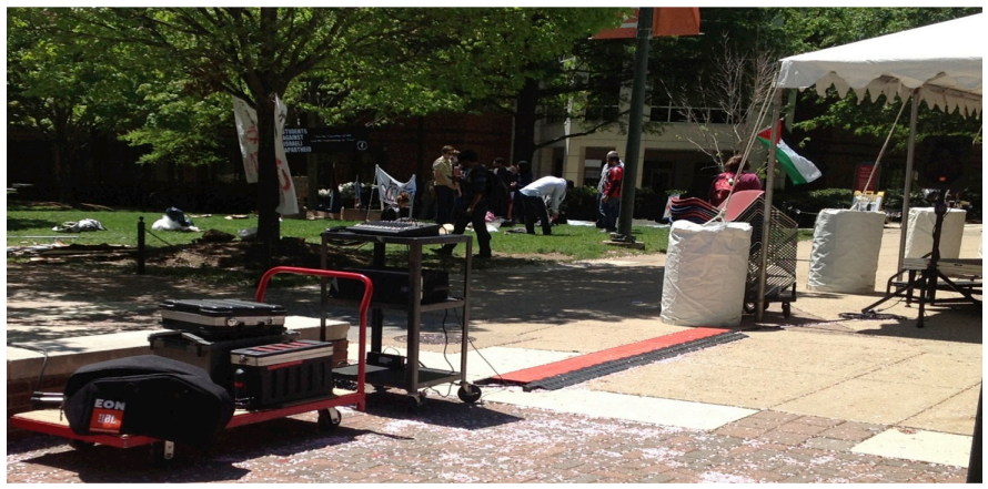
Figure 2. Example of a poor surface condition
