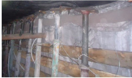
FIGURE 10: The effect of the filling body in the mold bag after solidification.
