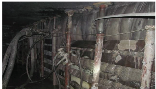
FIGURE 9: Mold bag filling completed.
