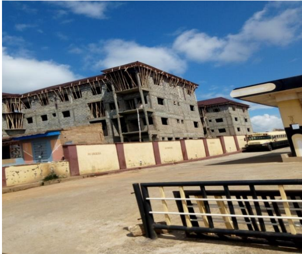
Plate 3: Land Use Conversion to a Hostel Close to Filling Station at MFM Junction, Tanke, Ilorin Source: Author's Field Survey (2019)
