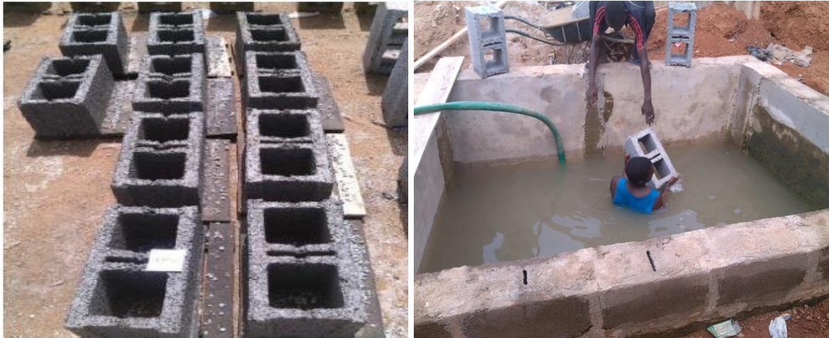
Fig. 4: Manufactured and Curing of Masonry Hollow Concrete Blocks.
