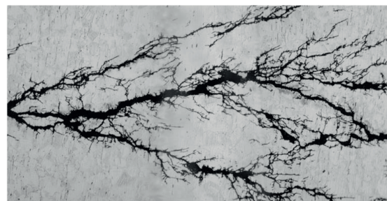
Fig. 2. Internal structure of the SC crack (after destructive evaluation)
