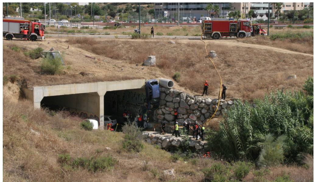
(a) View of the entrance of the tunnels
