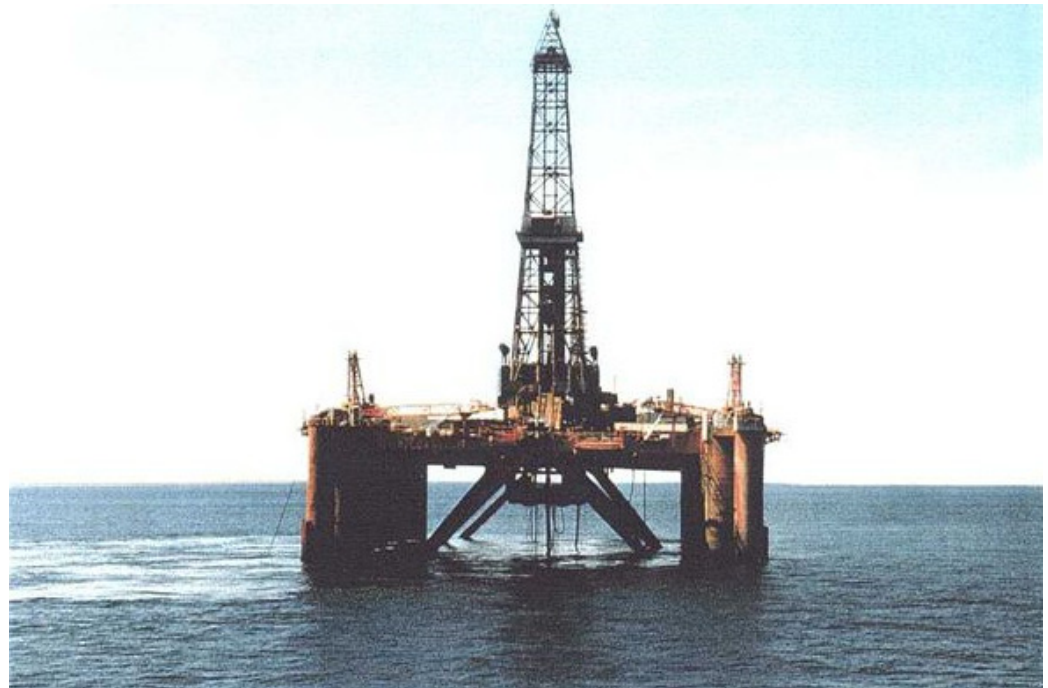
Figure 41. An offshore platform in the Andaman Sea, tilted by 3^\circ during the passage of an internal wave. Much of the tilt is into the plane of the image.
