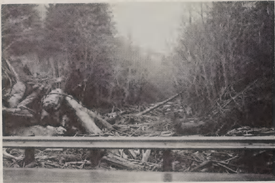
Mile 7 on the Wilson Highway--Debris-choked tributary stream.
