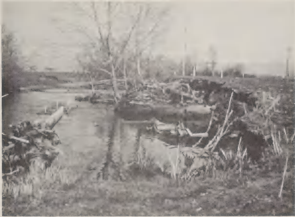
Channel bank erosion--Agricultural land.
