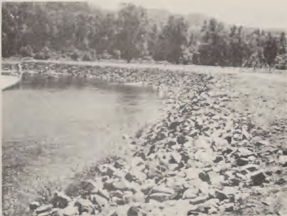
Riprap installation--Agricultural land.
