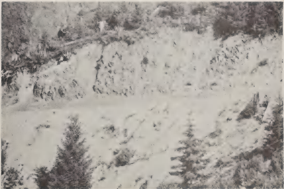
Roadside erosion--Forest lands.
