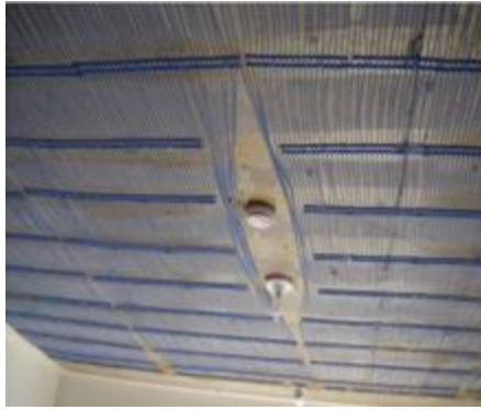
Figure 6 A photo taken during Installation of capillary tubes to the ceiling
