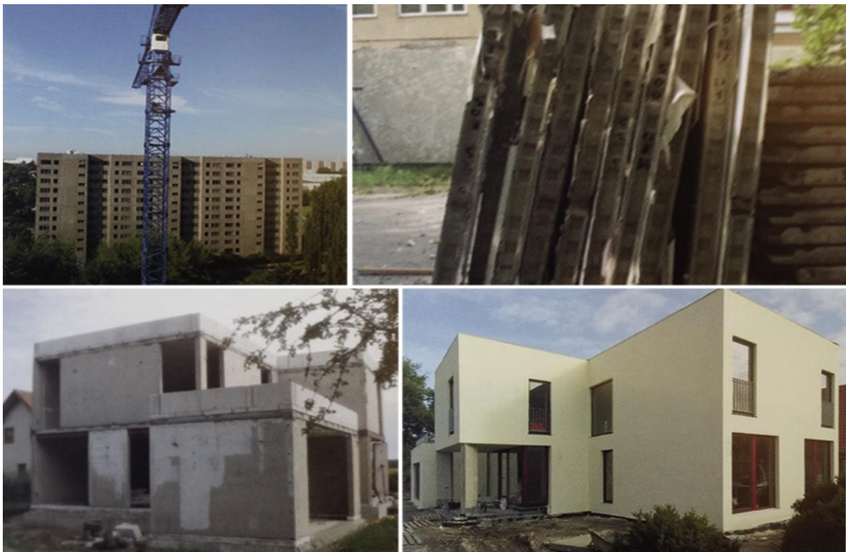
Figure 2 Reuse of precast concrete slabs and panels for new housing construction in Mehrow, near Berlin (source: Stacey, 2011)
