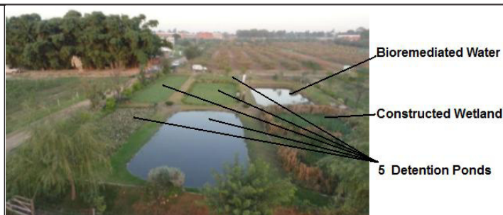
Fig 5. Five interconnected detention ponds precede constructed wetlands at the he Bioremediation Garden, National Agricultural Research Center, Islamabad.
