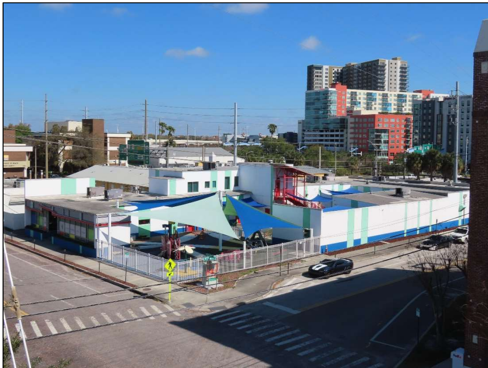
Figure 8.6: Carlton Academy Day School (8HI15085), c. 1946, located at 205 N Brush Street, considered National Register-eligible, facing Northeast
