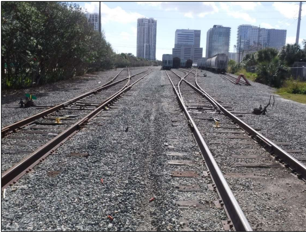
Figure 8.1: Existing Railway Corridor Containing Associated Gravel Ballast, Tracks, and Ties, Preventing Subsurface Testing Within Pond C, Facing South
