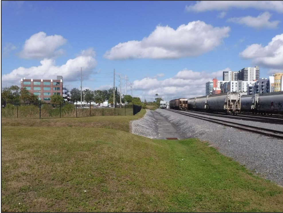
Figure 8.2: Modified Embankment, Drainage Ditch, and Existing Railway Corridor Containing Associated Gravel Ballast, Tracks, and Ties, Preventing Subsurface Testing Within Pond D, Facing North
