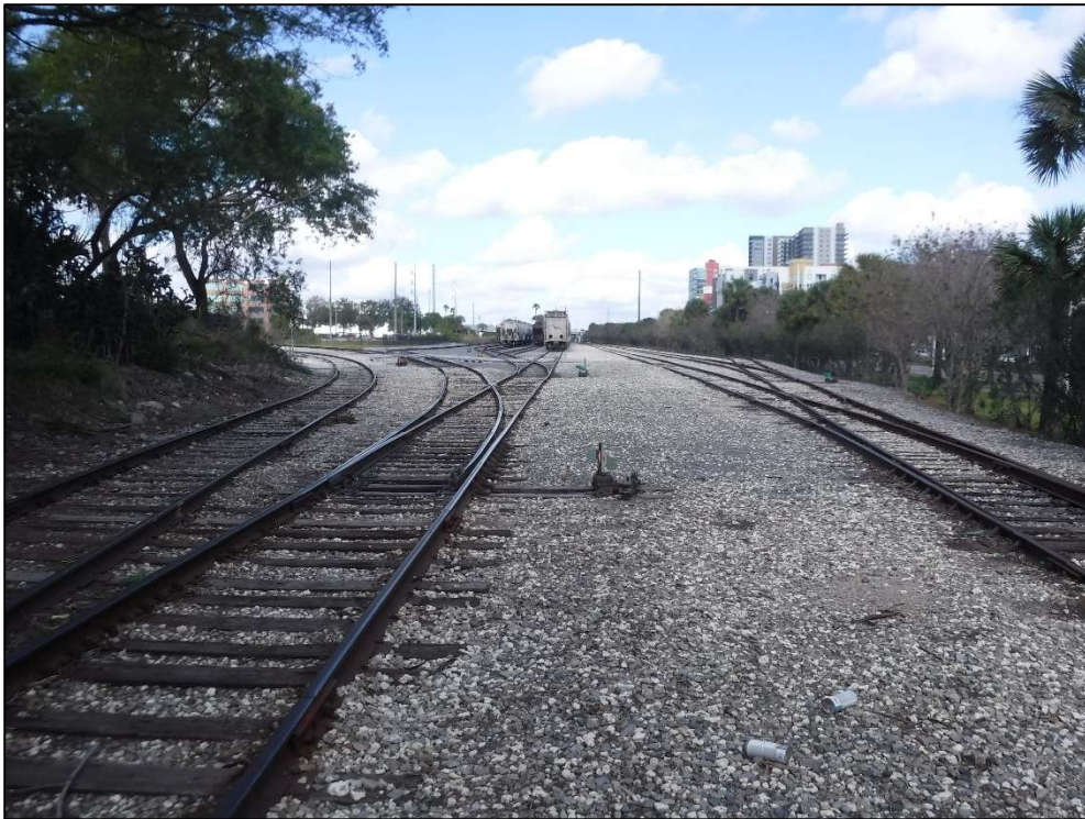
Figure 8.3: Existing Railway Corridor Containing Associated Gravel Ballast, Tracks, and Ties, Preventing Subsurface Testing Within Pond E, Facing North
