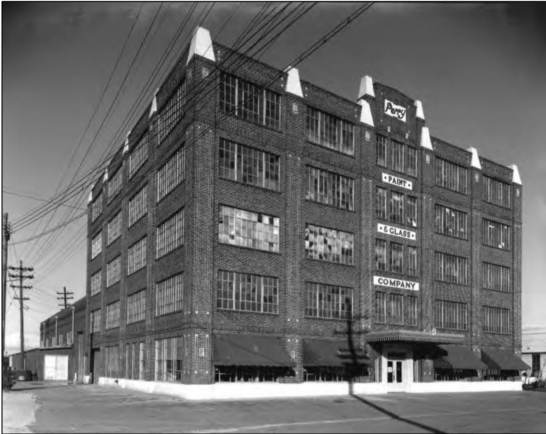
Figure 5: A 1948 photograph of the Perry Paint and Glass Company Building (8HI685), located at 109 N Brush Street (Courtesy, Tampa- Hillsborough County Public Library System)
