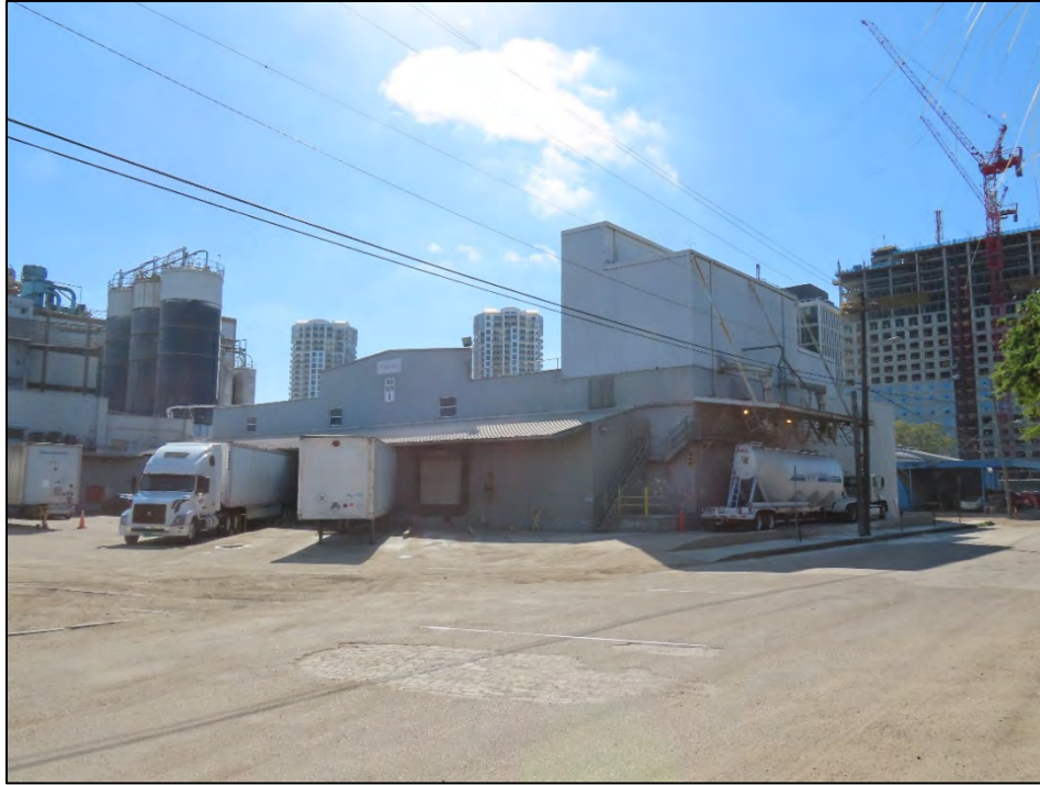
Figure 2: Ardent Mills (8HI15084), c. 1946, located at 110 S Nebraska Avenue, considered National Register-eligible, facing Southeast
