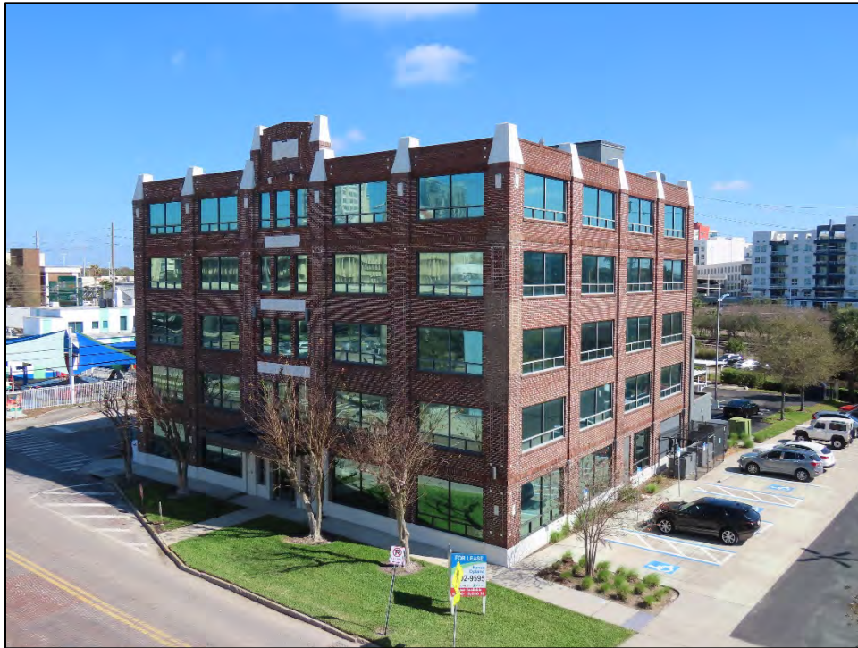
Figure 10.22: The Perry Paint and Glass Company Building (8HI685), c. 1928, located at 109 N Brush Street, considered National Register-eligible, facing Northeast
