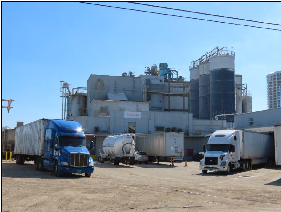
Figure 3: Ardent Mills (8HI15084), c. 1946, located at 110 S Nebraska Avenue, considered National Register-eligible, facing East
