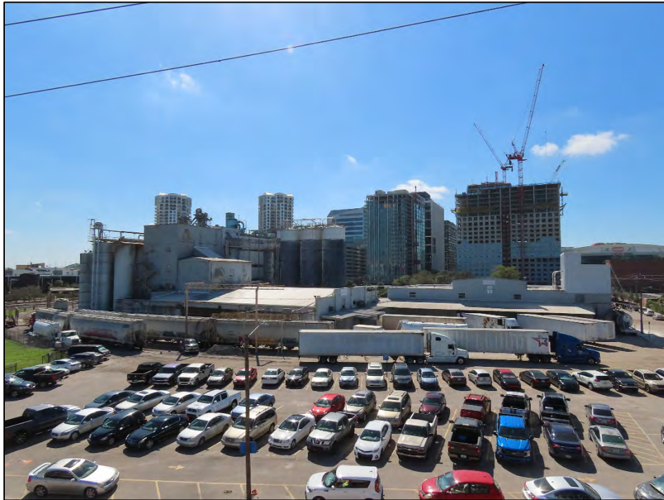
Figure 10.32: Ardent Mills (8HI15084), c. 1946, located at 110 S Nebraska Avenue, considered National Register-eligible, facing South
