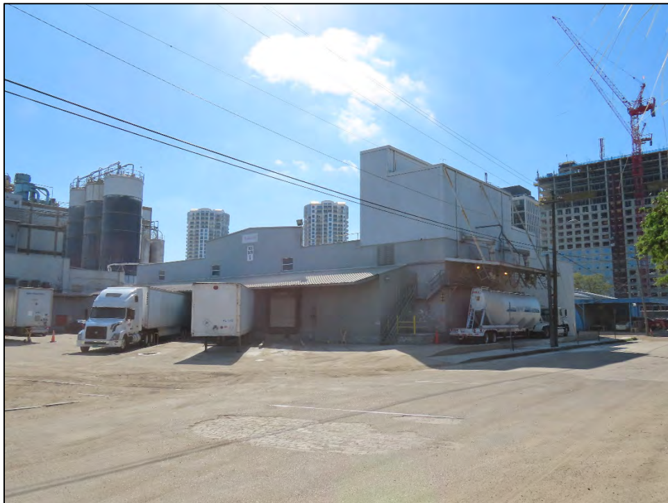
Figure 10.33: Ardent Mills (8HI15084), c. 1946, located at 110 S Nebraska Avenue, considered National Register-eligible, facing Southeast
