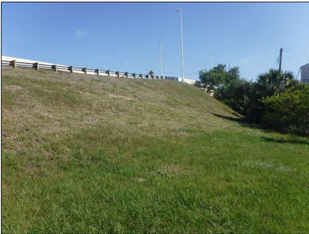
Figure 10.6: View of Bermed Ramp for Exit from the Selmon Expressway
