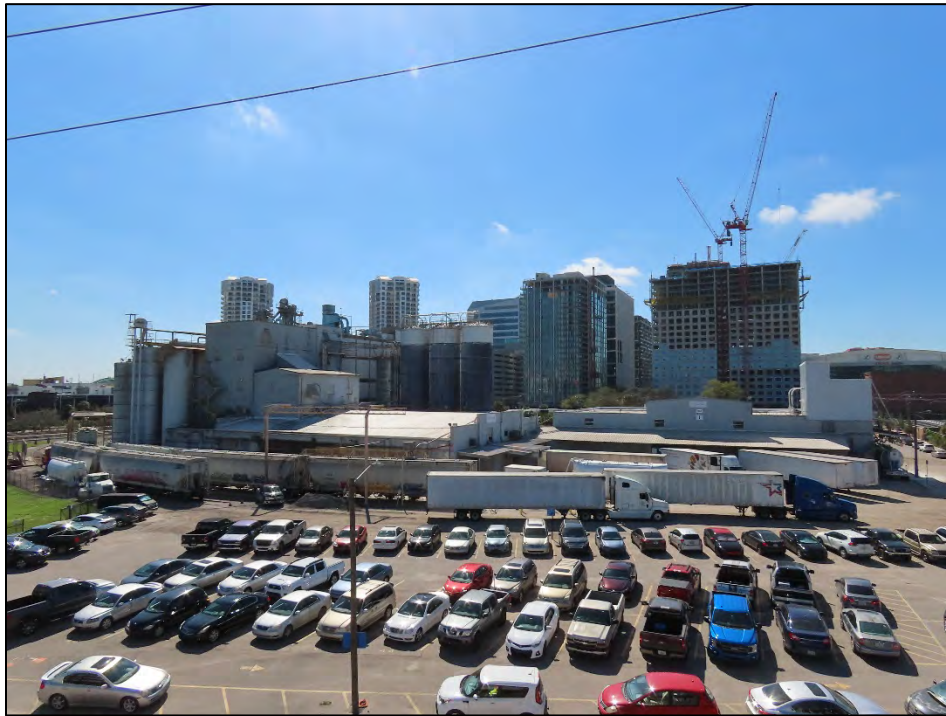
Figure 1: Ardent Mills (8HI15084), c. 1946, located at 110 S Nebraska Avenue, considered National Register-eligible, facing South
