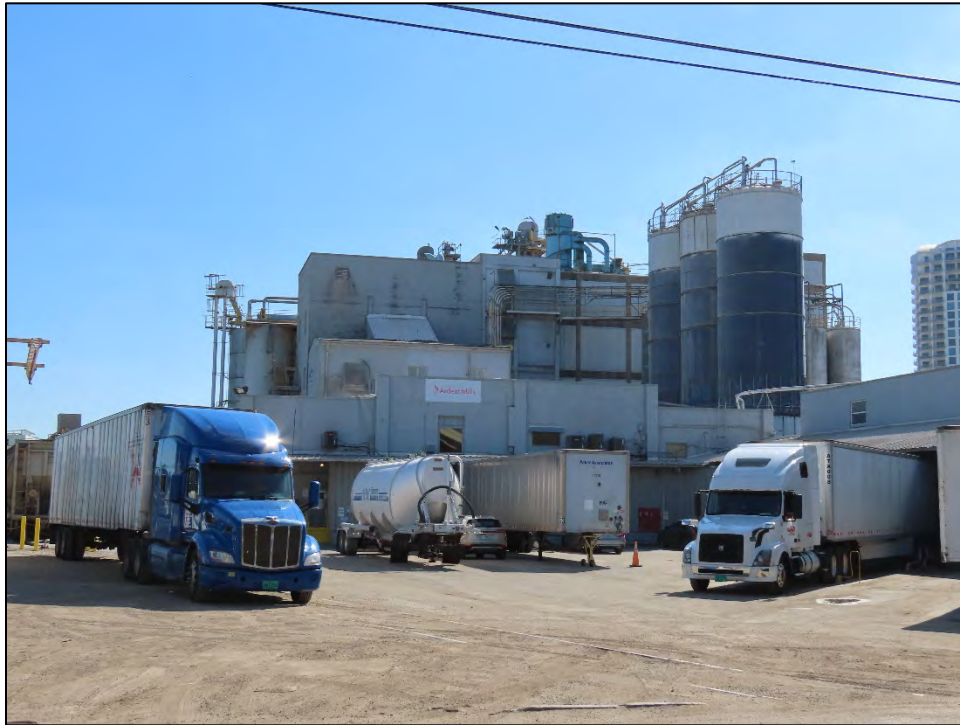
Figure 10.34: Ardent Mills (8HI15084), c. 1946, located at 110 S Nebraska Avenue, considered National Register-eligible, facing East
