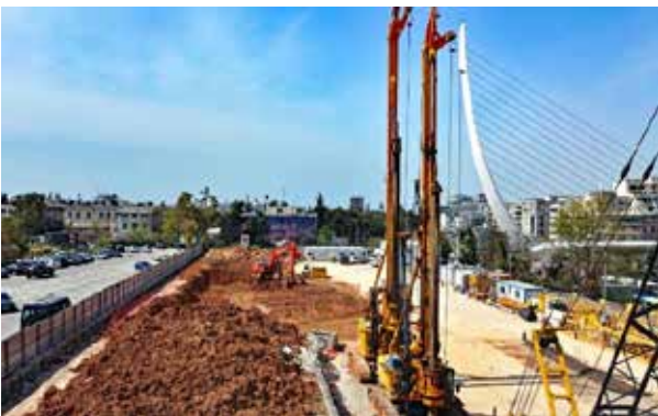
Katehaki Shaft – boring of piles for retaining walls
