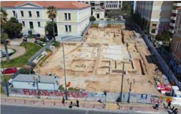
Akademia Station preparatory works
