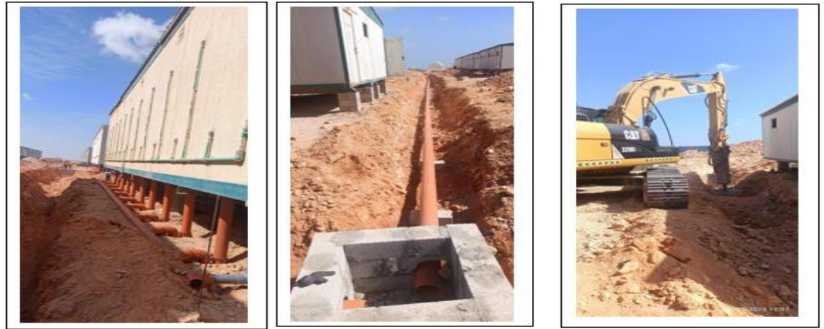
Underground work & plumbing under progress
