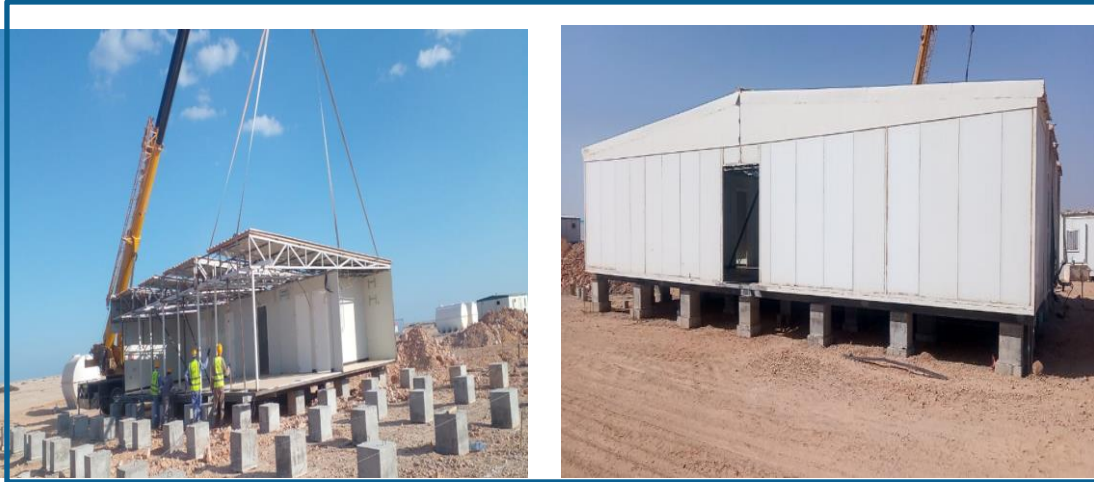
Site office Installation
