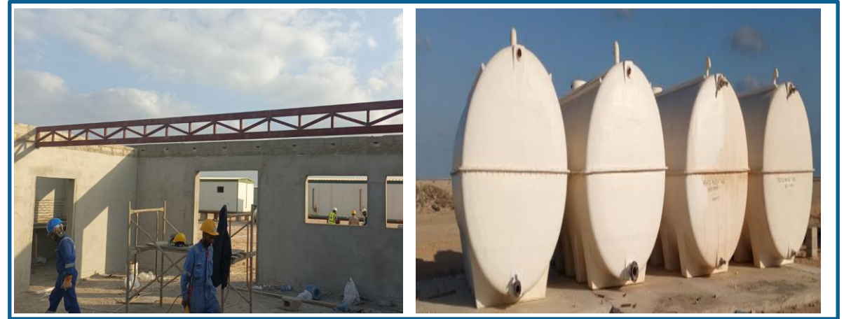
Kitchen block & Water Tank
