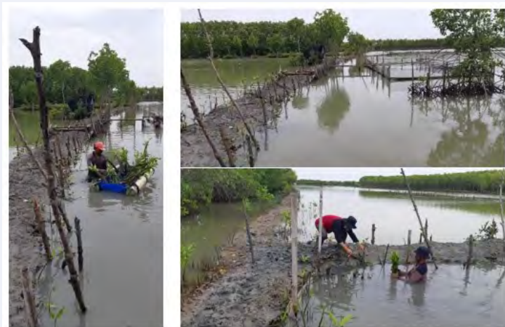
FIGURE 12. Demonstration site development.
