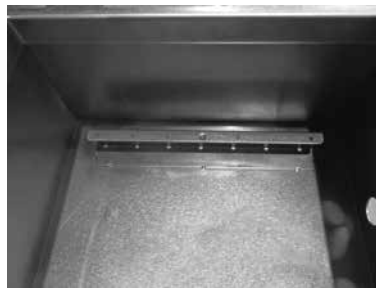
Support for DIN rail without mounting plate
