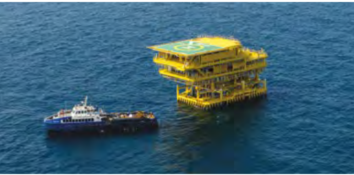
▲ Newly-installed wellhead platform Arabian Gulf
