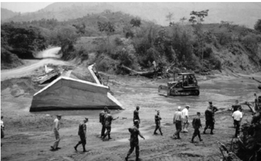
An ARNG bulldozer installs culverts over Rio San Juan in Honduras during Exercise New Horizons.
