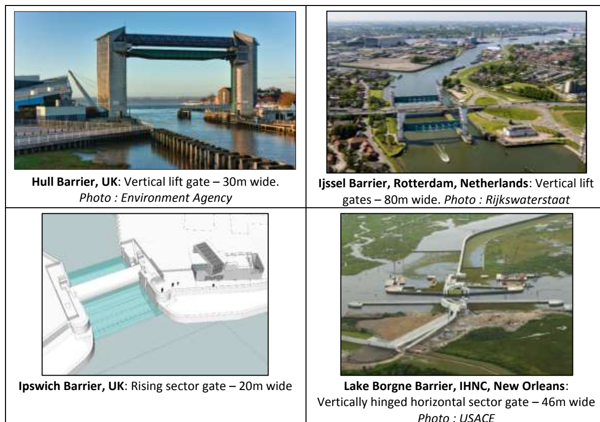
Figure 4.2 Example barriers and gates
