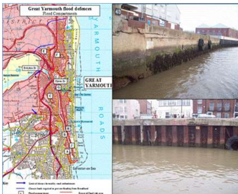
Figure 2.2 Great Yarmouth flood compartments and tidal walls
