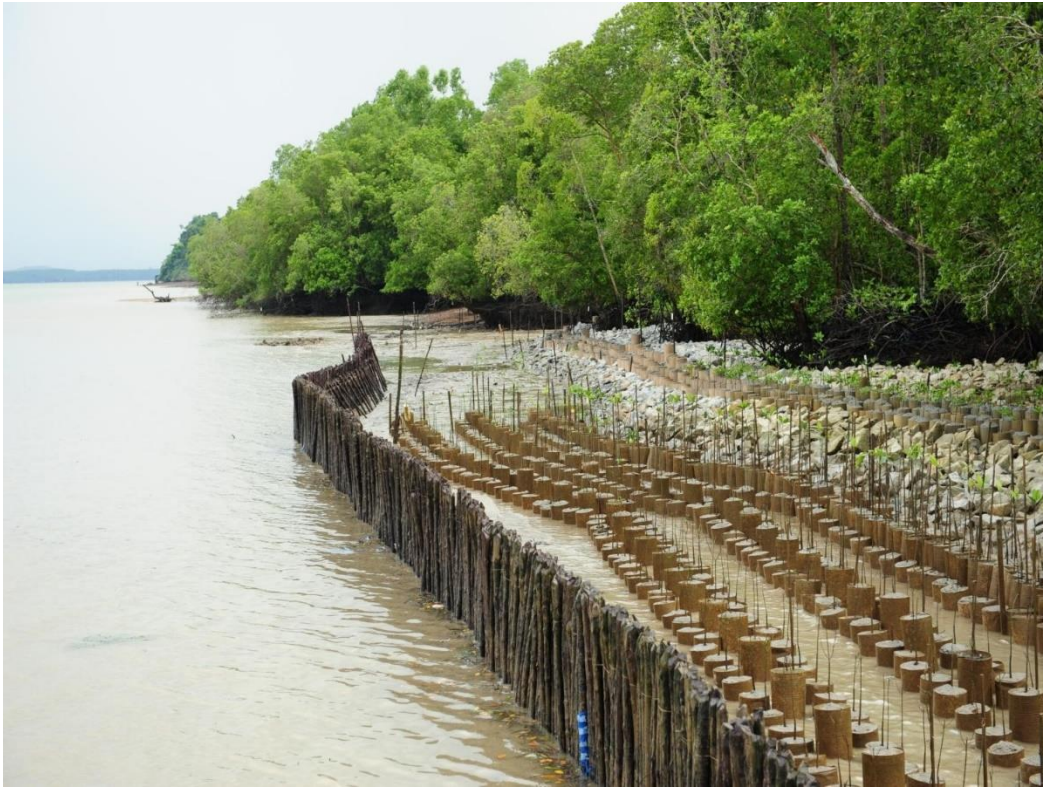
Figure 5 Restored section of the shore on Pulau Tekong Island (Source: NParks)
