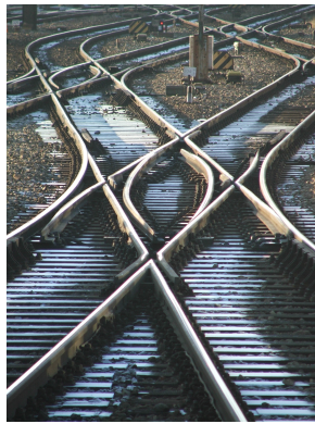
Fig. 6: Double slip switch at Munich Central Station by Láczy [38] published under a CC BY-SA 2.0 license
