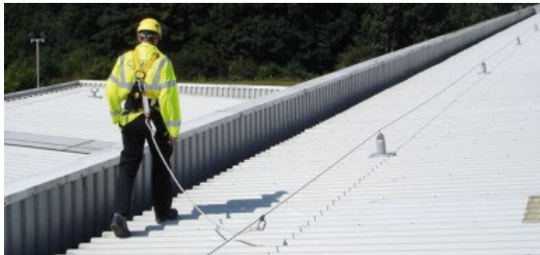
Fall arrest system on horizontal lifeline
