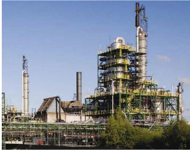
Figure 4.3.2. BioMCN Biomethanol Plant
