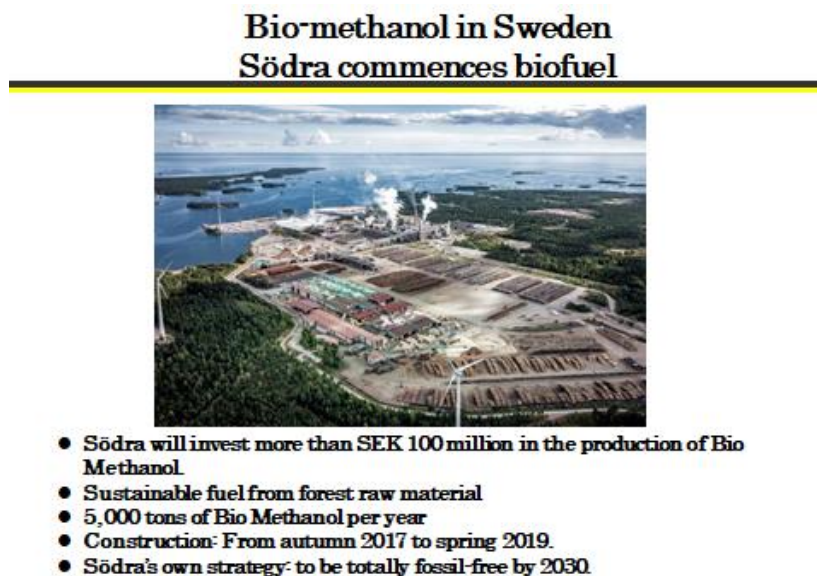
Figure 4.3.7. Södra Biomethanol Plant in Sweden
