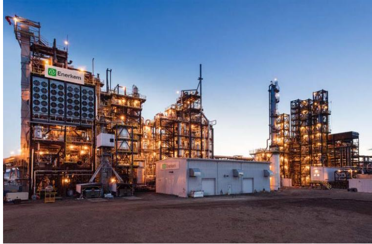
Figure 4.3.4. Enerkem Alberta Waste-to-Biofuel Plant
