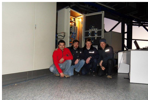
Figure 3.196. The Paranal and Garching UT1 to E-ELT standards dome team following the successful installation.
