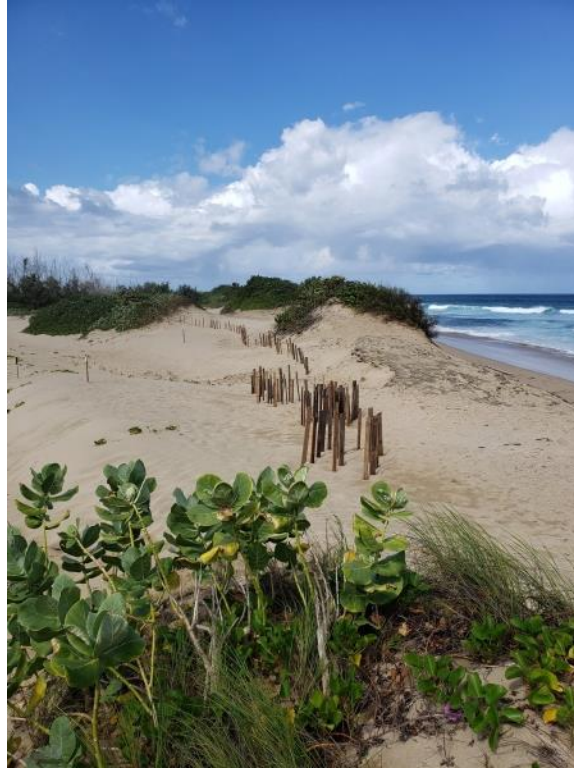
Figure 0-16: Sand-trapping devices used by Vida Marina (NOAA)
