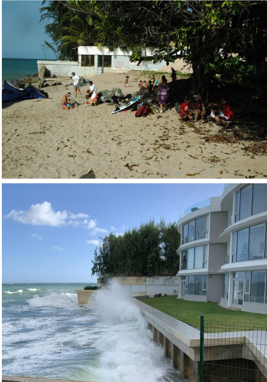
Figure 0-2: Top: former sandy beach at Punta Las Marias in San Juan, Puerto Rico. Bottom: same site after the construction of a steel sheet pile bulkhead with a concrete cap to manage swells and coastal flooding. The bulkhead exacerbated to the loss of sand, further coastal erosion at the toe of the structure, reduced public access, and the loss of recreational and ecological values once associated with this beach area (N. Pérez, used with permission).
